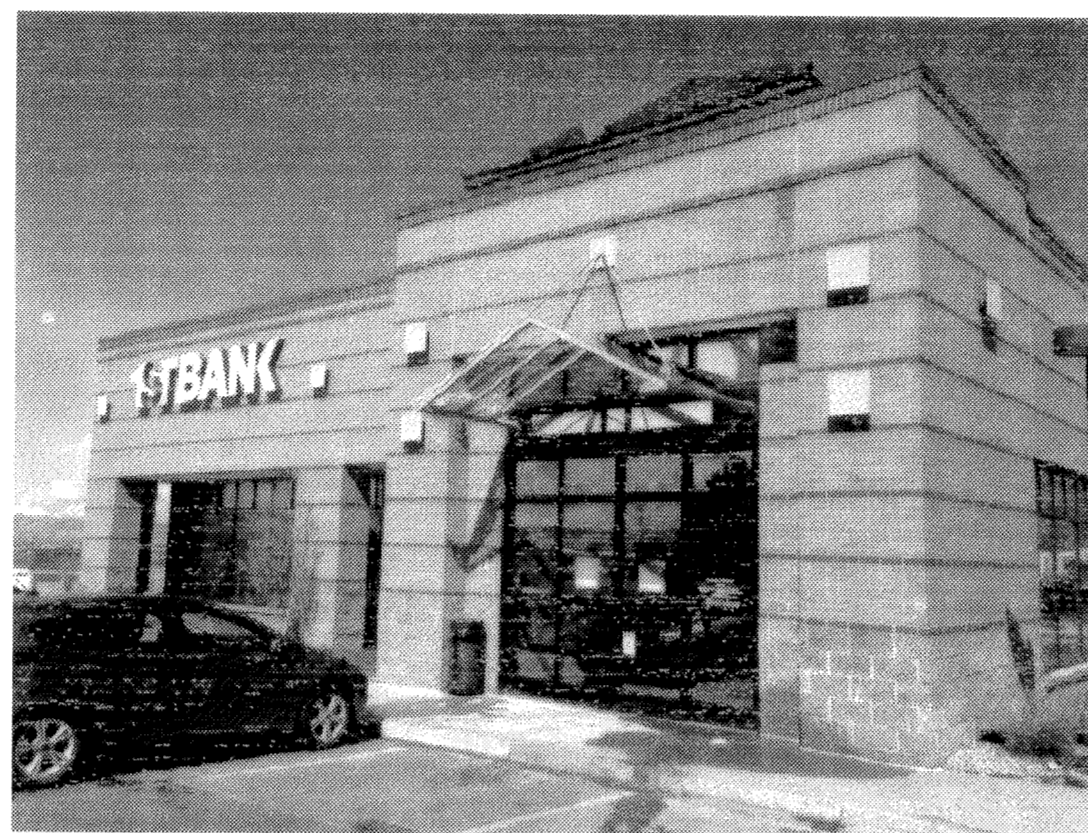
REFERENCE PHOTO: EXISTING SCONCES AND POLE FIXTURE STYLES (EXISTING TO REMAIN)
