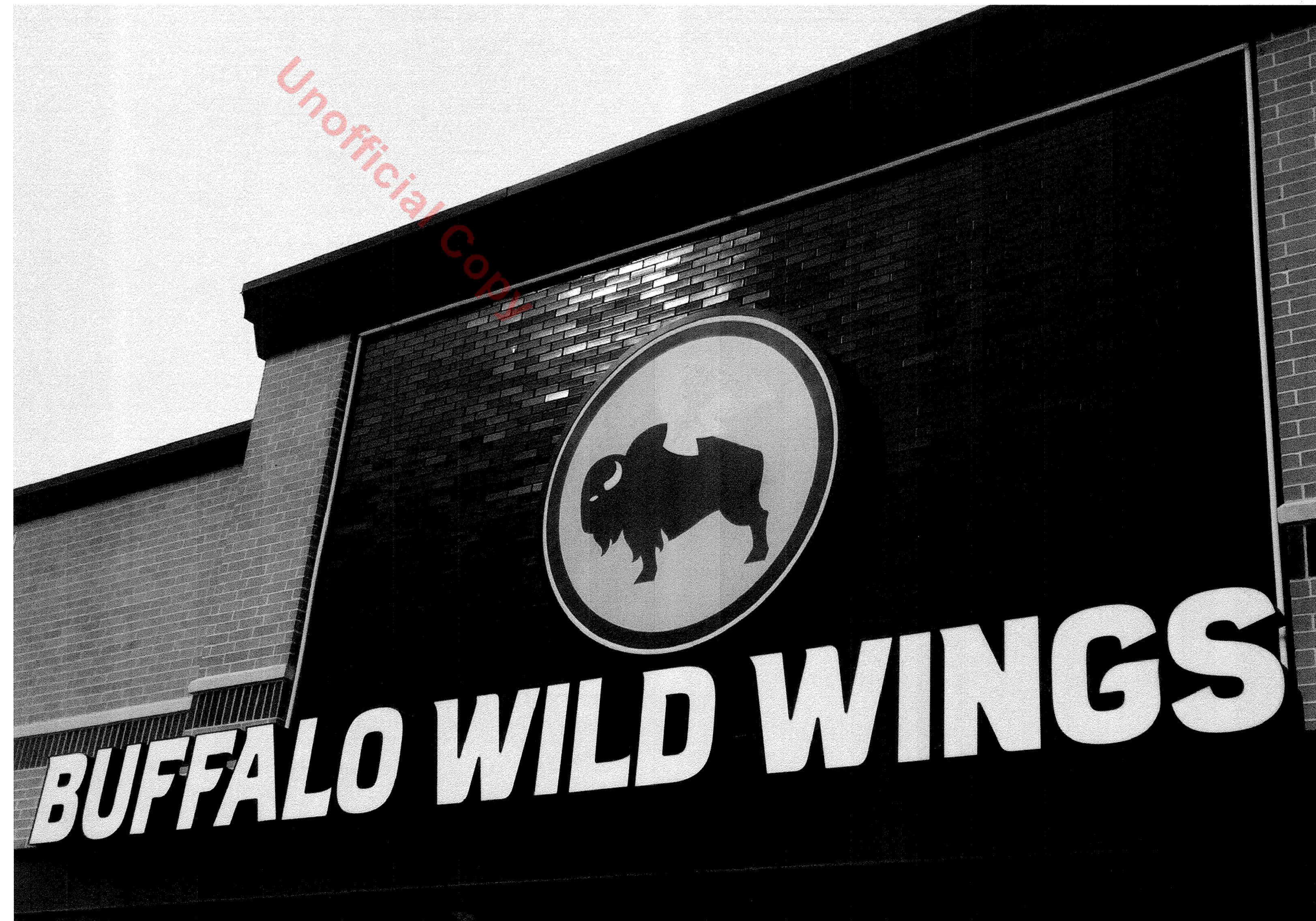
2. REFERENCE PHOTO FROM SIMILAR PROJECT: FIBER CEMENT PANELS - NICHIIA PLYMOUTH BRICK CRIMSON EPF151F, PAINTED GLOSSY BLACK
