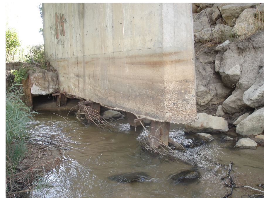
Exhibit IV-13: Pier group underneath South Wilcox Bridge and East Plum Creek
