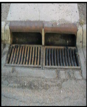
Directional Cast Vane Grate
