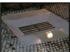
CDOT Type D Inlet Parallel (Flat & Depressed)
