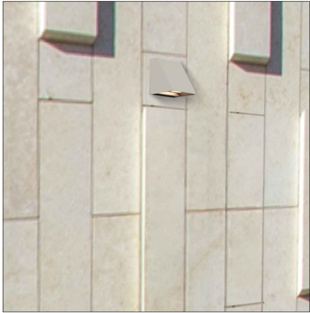
9 Exterior Wall Mounted Lighting
