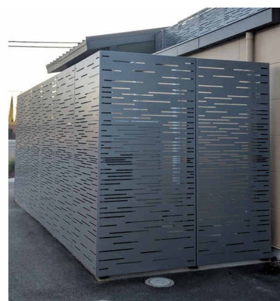
6 MECHANICAL SCREENING FOR ROOF EQUIPMENT 1/8" = 1'-0"
