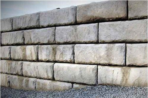
REDI-ROCK GRAVITY WALL WALL TO BE GRAY OR SIMILAR NATURAL COLOR
