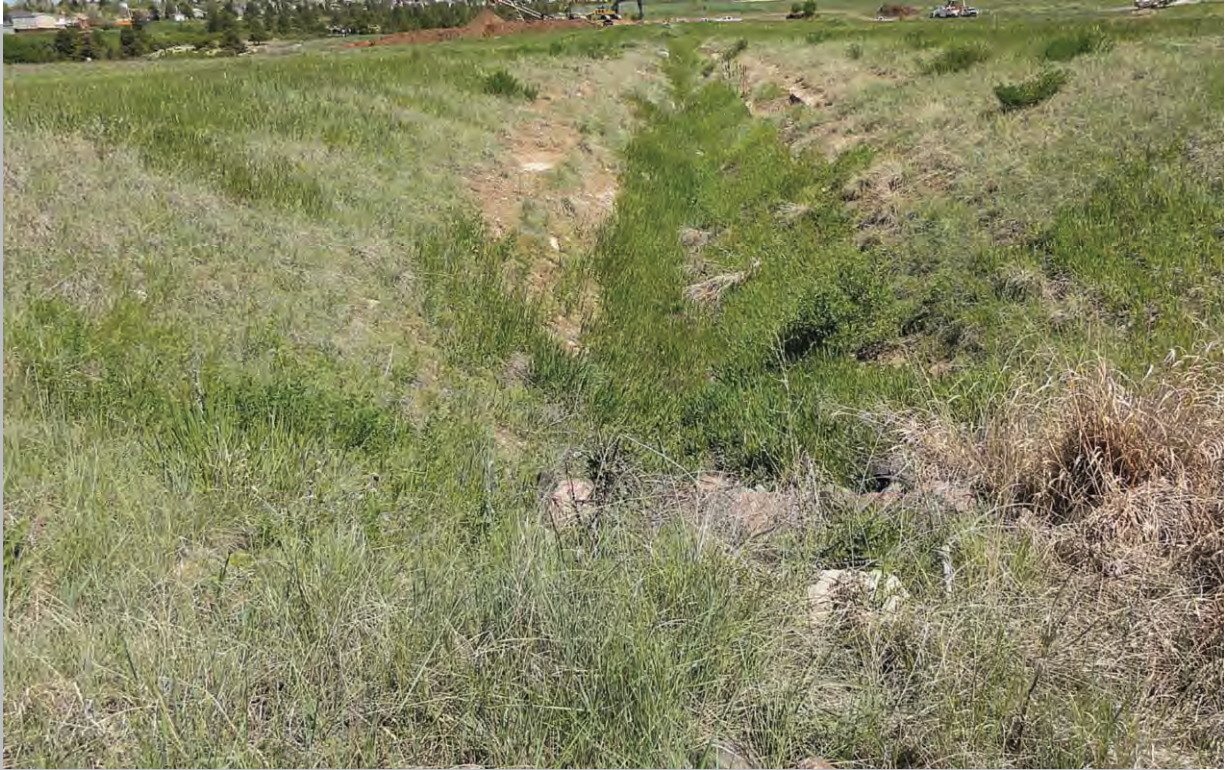
Photo 7 - View of the shallow ditch at the northeast corner of the property.
