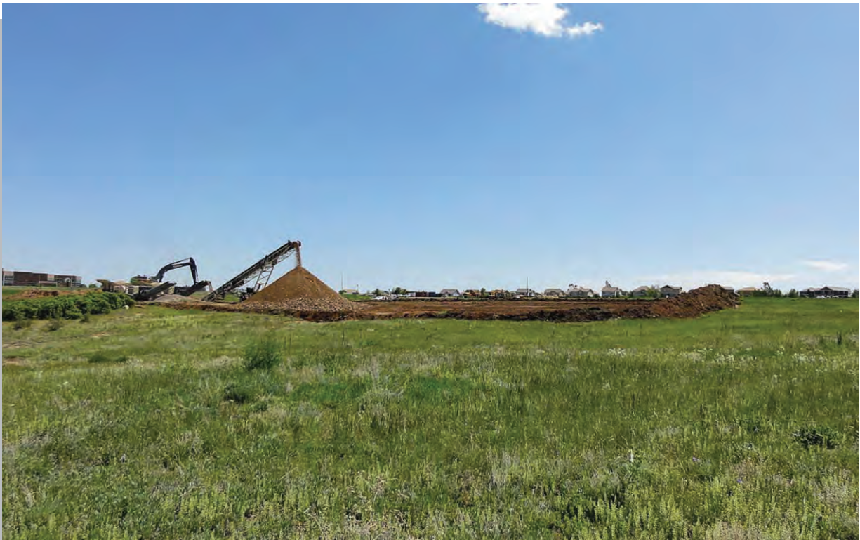
Photo 10 - View of the north adjoining property, vacant land under construction.
