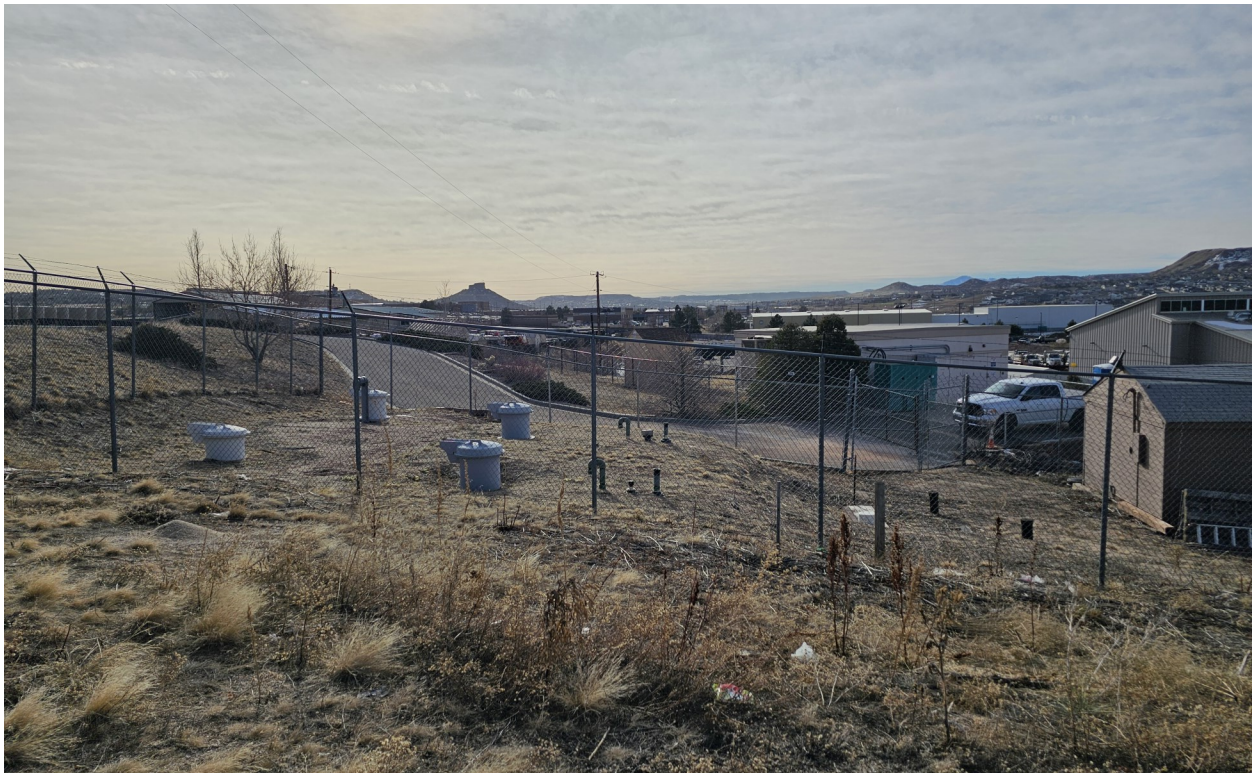
No. 14 | View of the Castleton Water and Sanitation District water taps
