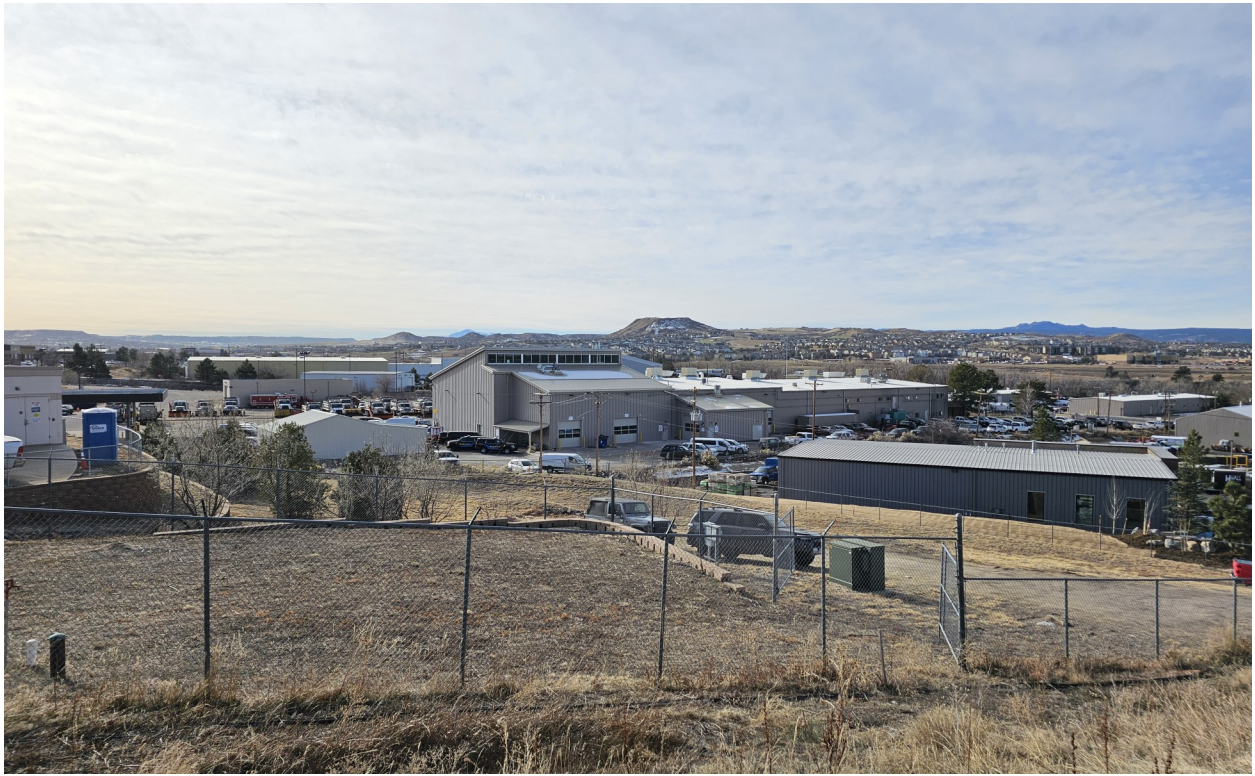
No. 13 | View of the southern Douglas County Maintenance Services Building
