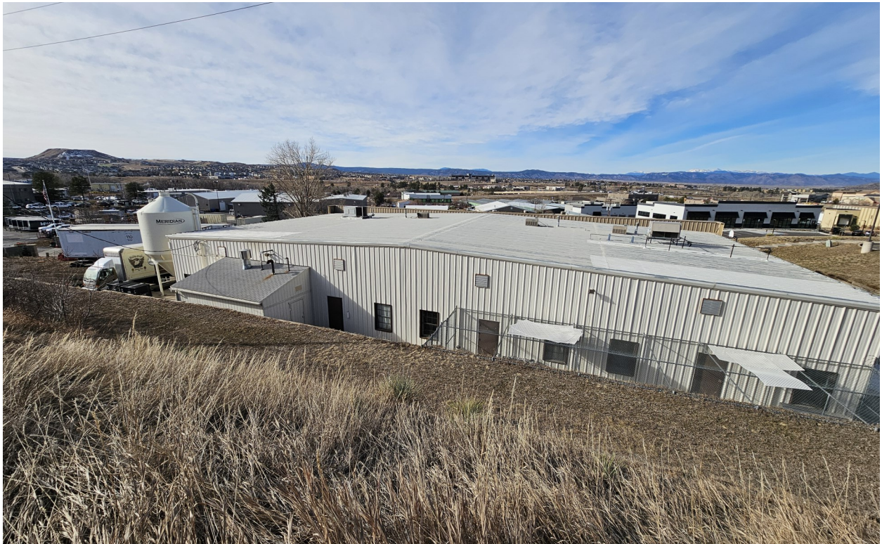
No. 15 View of the western Rockyard Brewing warehouse
