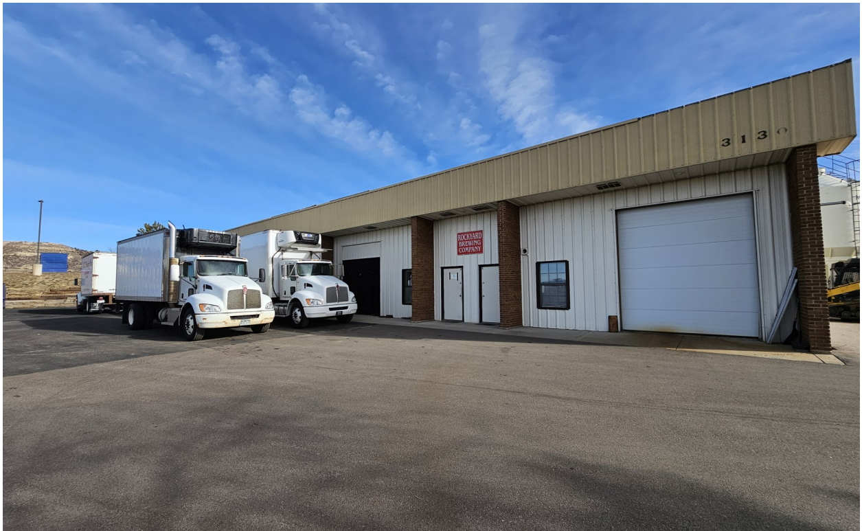
No. 16 Front view of the Rockyard Brewing Warehouse
