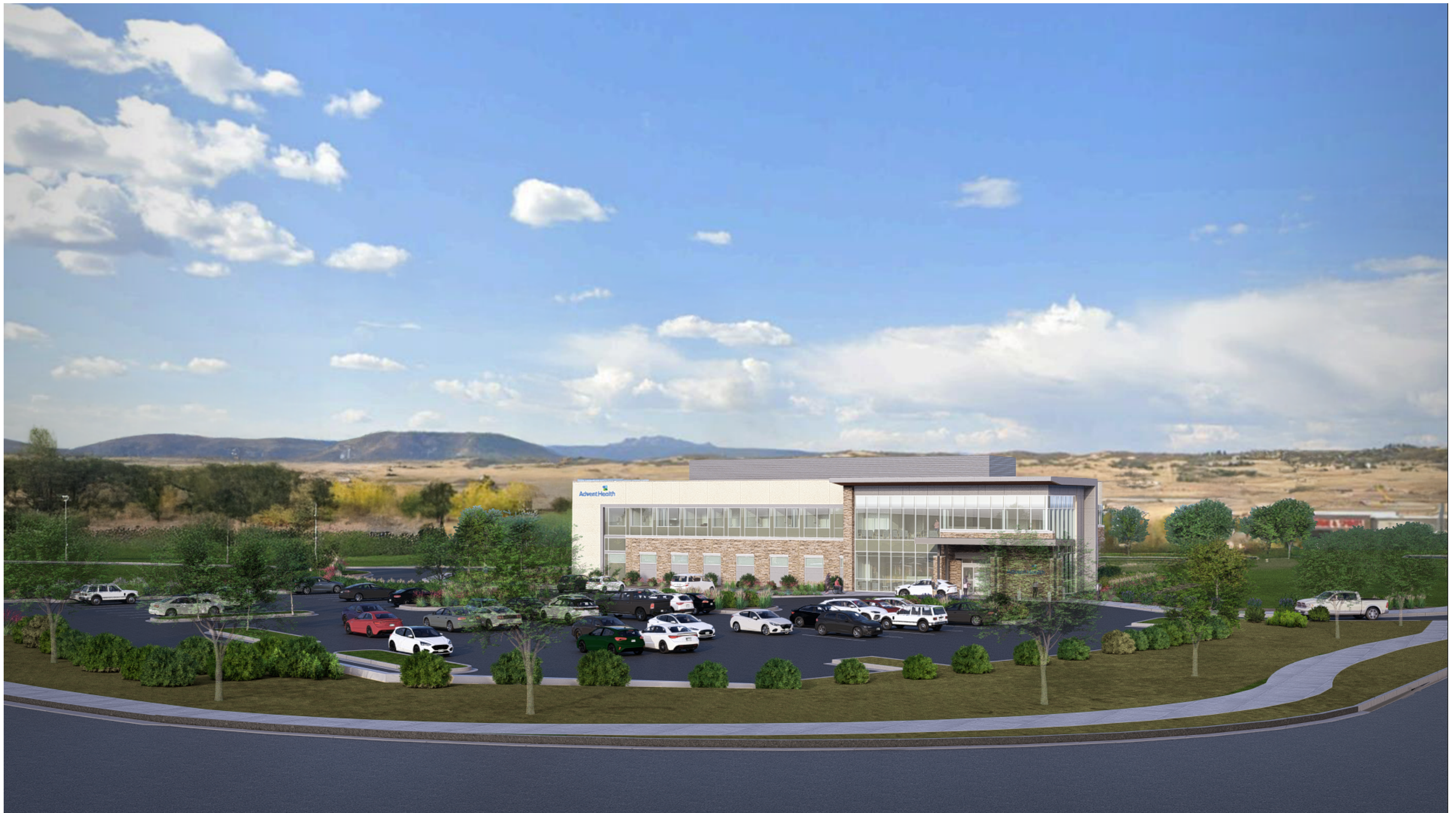
Street View from Roundabout
