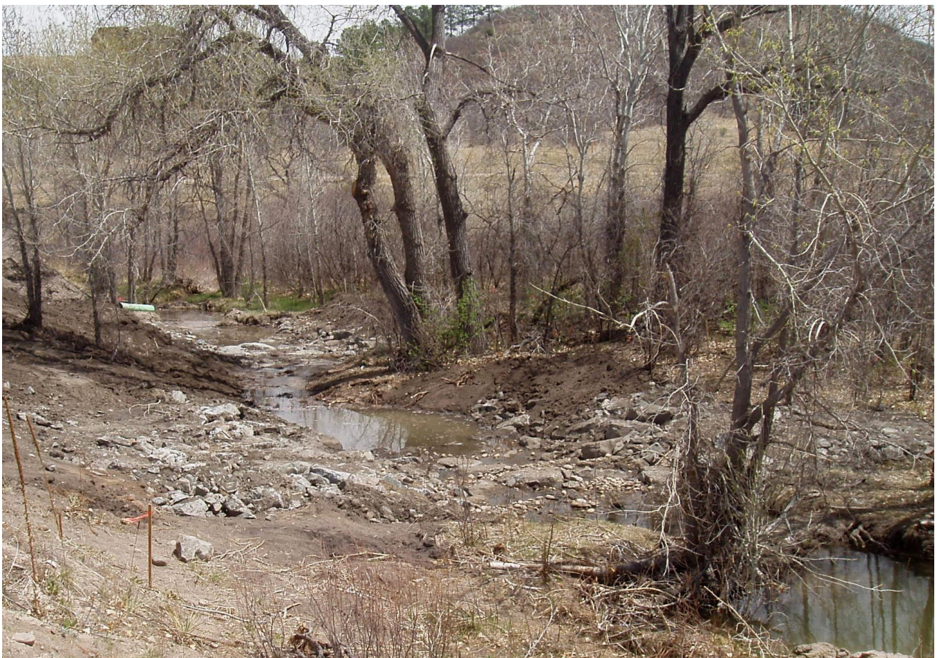
Boulder cascade drops being constructed at critical locations to protect the Gulch against major erosion while preserving existing riparian vegetation.
