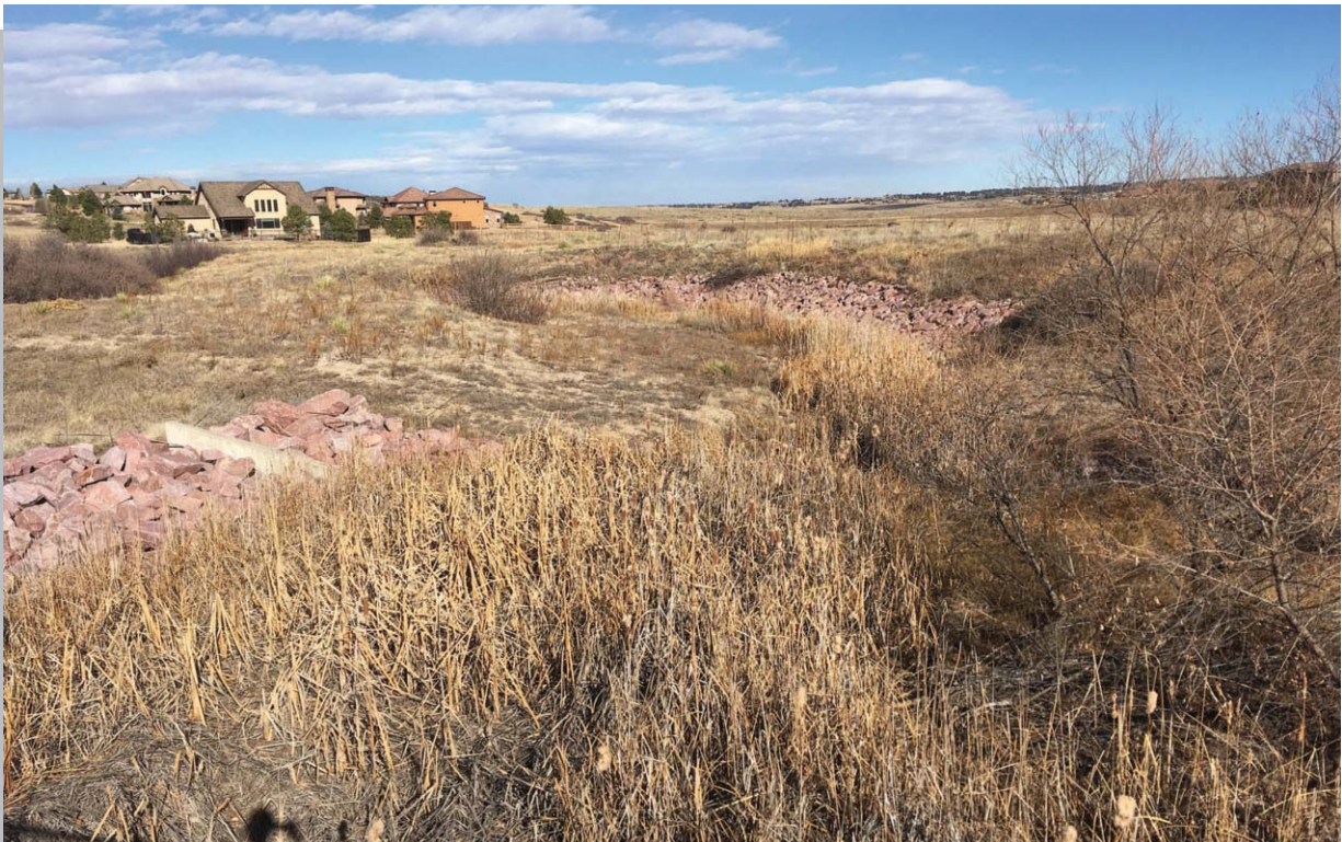
Photo 12 - The Scott Gulch channel downstream of Raintree Drive and upstream of the large irrigation pond on the Pradera Golf Course. View is to the northeast.
