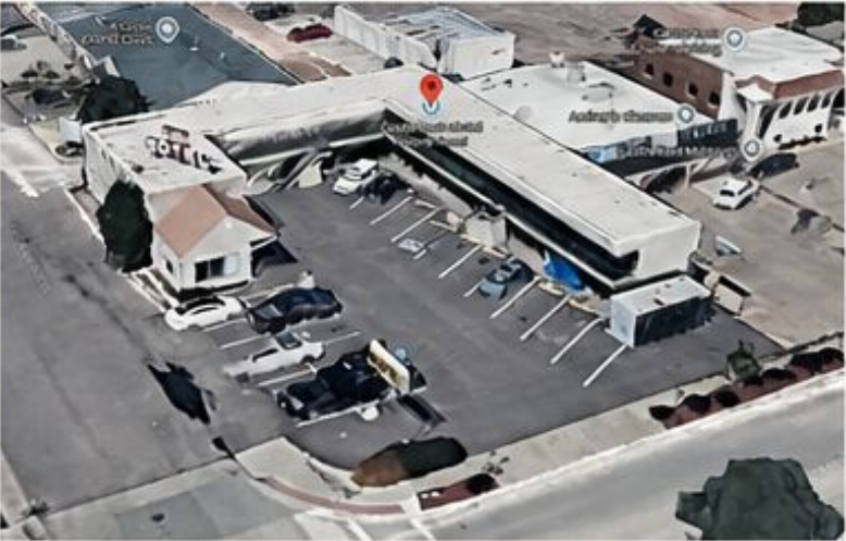
AERIAL VIEW FROM NORTHEAST
