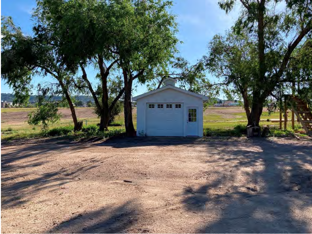
5DA2720 – Standing structure. Photo Number: JH1.019 Date: 6.29.20
