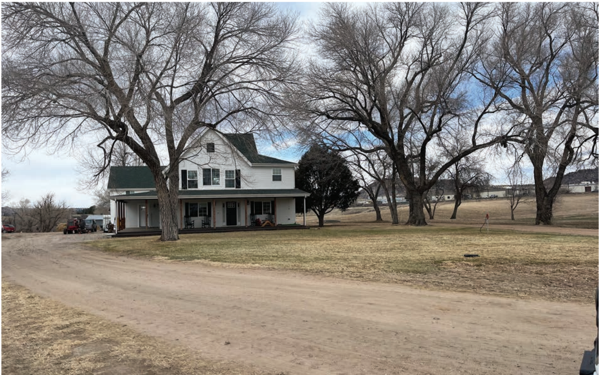
Photo 2 - Residence, blacksmith shop, and equipment storage yard in the western portion of the project area. View is north.
