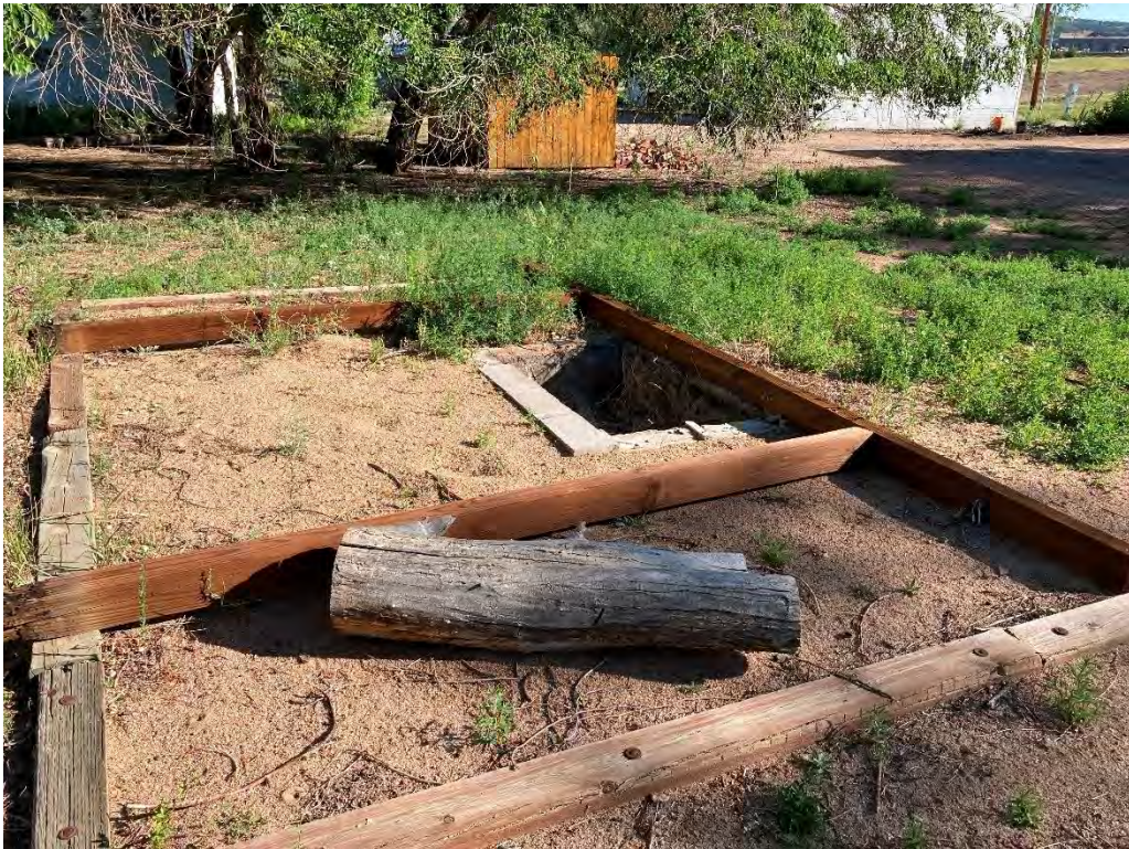
5DA2720 – Exposed foundation. Photo Number: JH1.16 Date: 6.29.20
