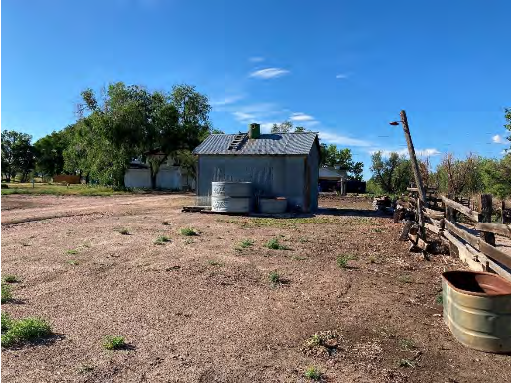
5DA2720 – Standing structure. Photo Number: JH1.23 Date: 6.29.20
