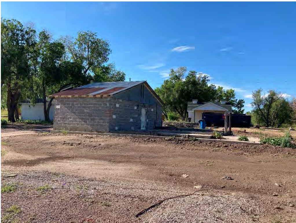
5DA2720 – Standing structures. Photo Number: JH1.22 Date: 6.29.20
