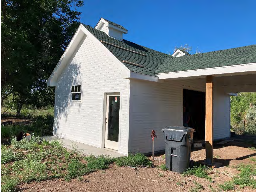
5DA2720 – Standing structure. Photo Number: JH1.017 Date: 6.29.20
