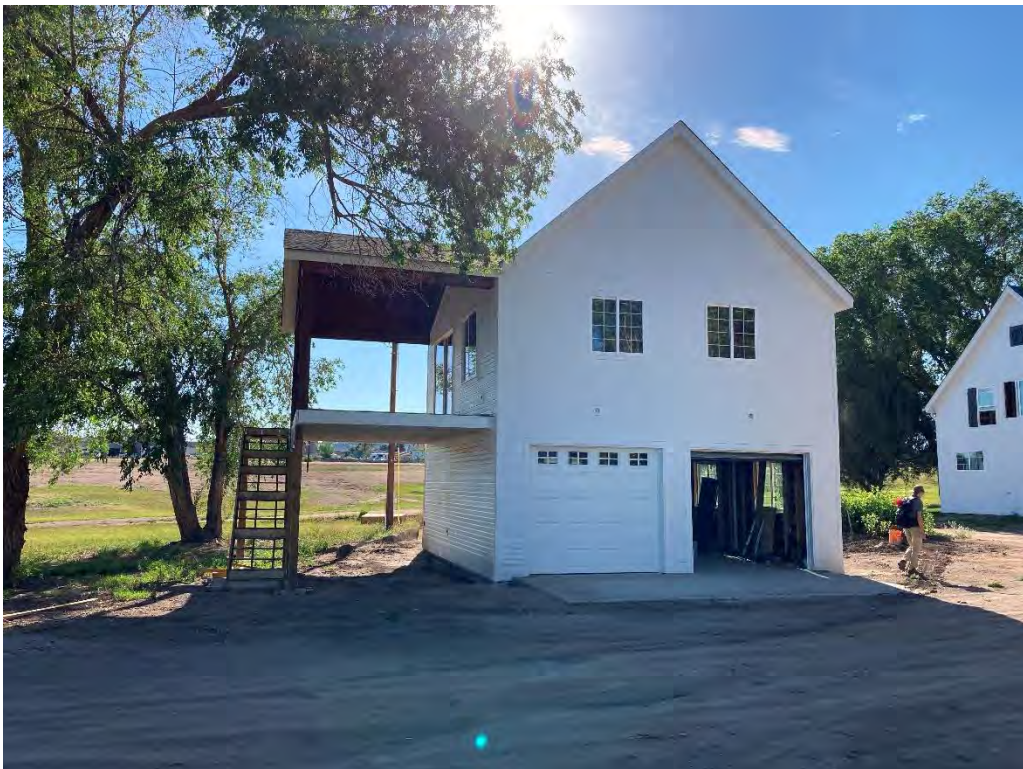
5DA2720 – Standing structure, view to the west. Photo Number: JH1.18 Date: 6.29.20
