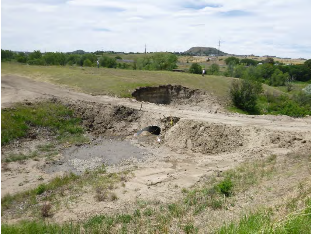
JH01 - Overview of ephemeral channel and modern bridge disturbance, view to the southwest. Photo Number: D3.107-0095 Date: 6.29.20
