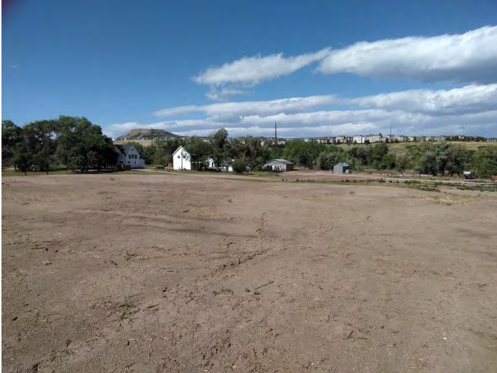
JH05 – Site overview facing site 5DA2720. View to the southeast. Photo Number: LT1.00004 Date: 6.30.20
