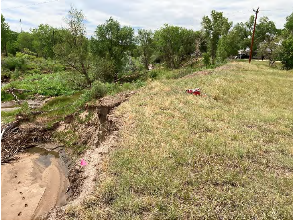
JH04 – Site overview facing Plum Creek and SDA2720, view to the northwest. Photo Number: JH1.28 Date: 6.30.20
