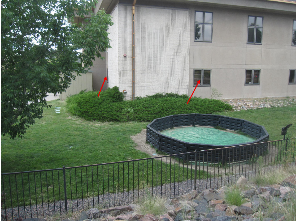
Photo 3. These junipers are an example of the risk posed being located beneath windows which may allow entry of a fire into the building.
