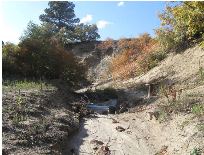
Exposed Utility Crossing in Reach 1 of the Omni Tributary
