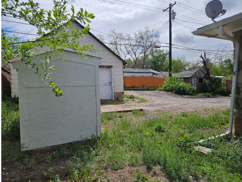
View of east side of the property, F2-4, view east (Roll 26-450, image 110107; Emily Wren; 5/22/2026)
