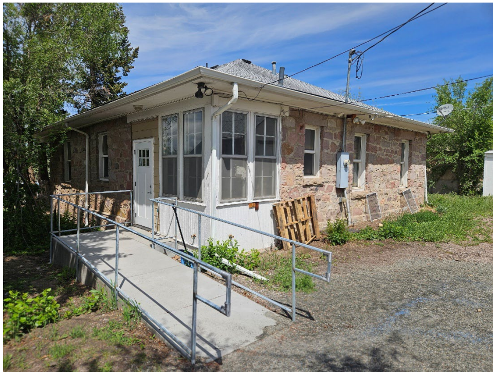
View of enclosed porch and ramp, view northwest (Roll 26-450, image 105208; Emily Wren; 5/22/2026)
