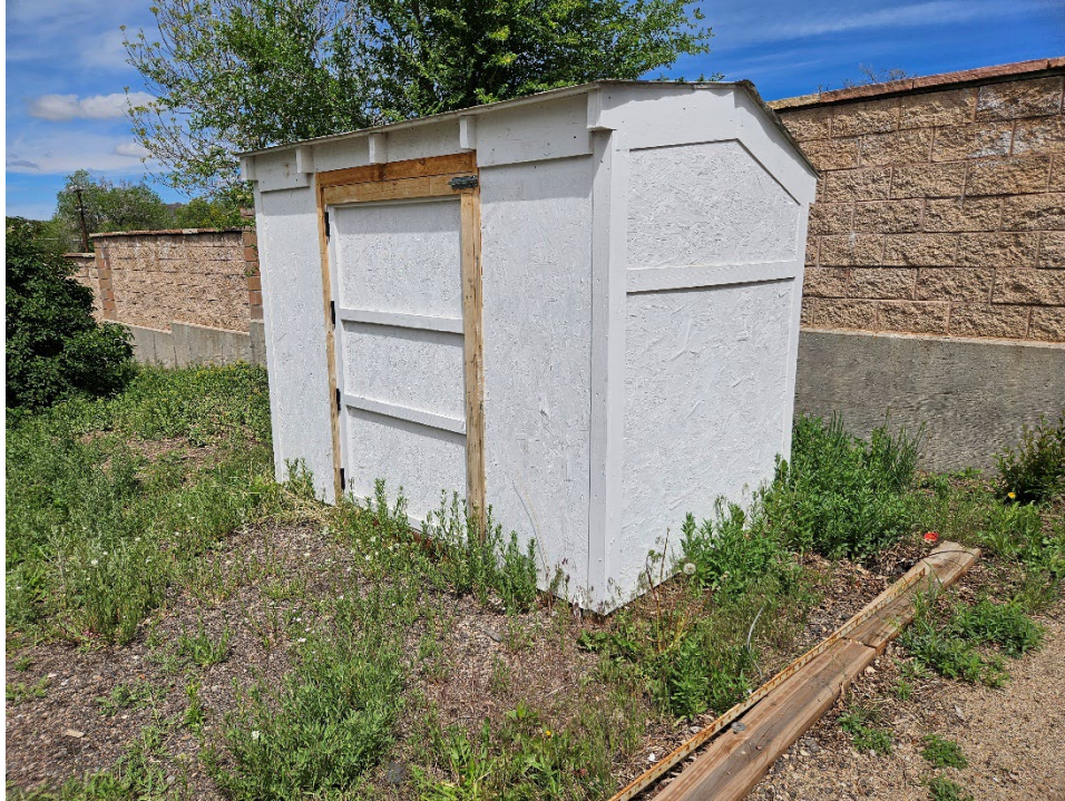
South and east elevations of F4 (shed), view northwest (Roll 26-450, image 110027; Emily Wren; 5/22/2026)
