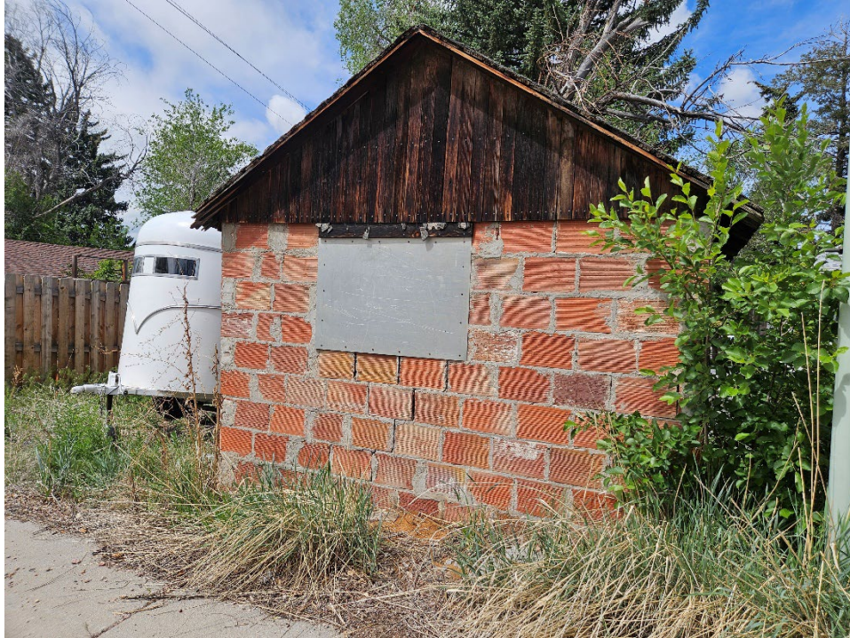
East elevation of F3 (shed), view west (Roll 26-450, image 105819; Emily Wren; 5/22/2026)
