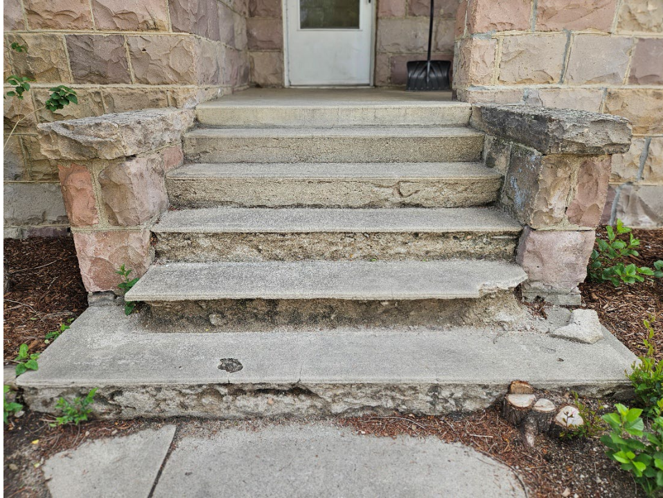
Close up of porch steps, view east (Roll 26-450, image 105335; Emily Wren; 5/22/2026)
