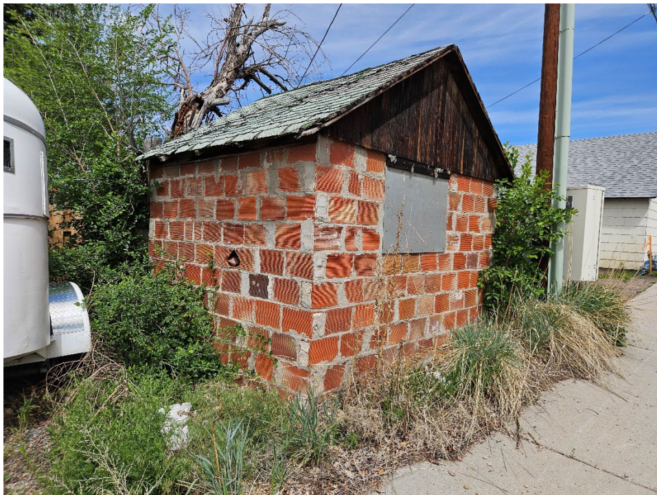
South and east elevations of F3 (shed), view northwest (Roll 26-450, image 105826; Emily Wren; 5/22/2026)
