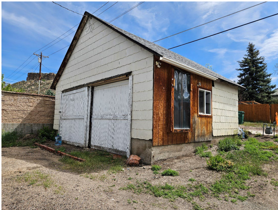
West and south elevations of F2 (garage), view northeast (Roll 26-450, image 105859; Emily Wren; 5/22/2026)
