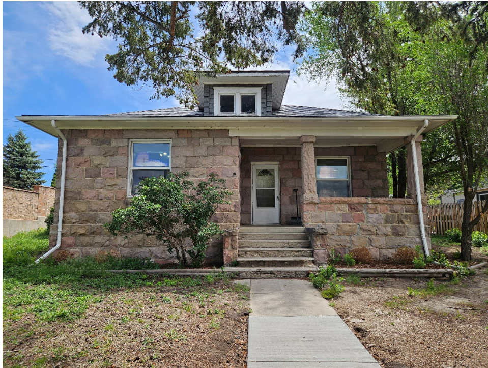
Primary (west) elevation of the residence, view east (Roll 26-450, image 110136; Emily Wren; 5/22/2026)
