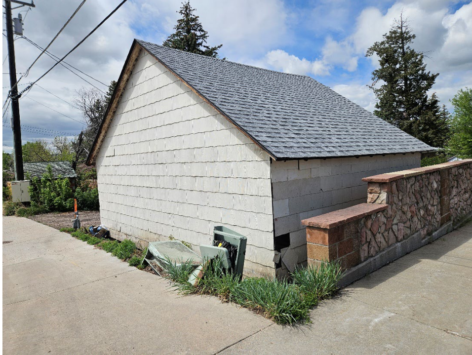
East and north elevations of F2 (garage), view southwest (Roll 26-450, image 105939; Emily Wren; 5/22/2026)
