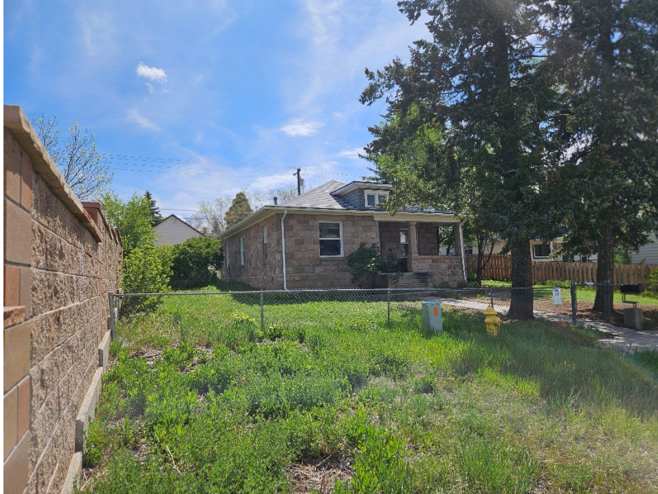
View of property from northwest corner, view east (Roll 26-450, image 104932; Emily Wren; 5/22/2026)
