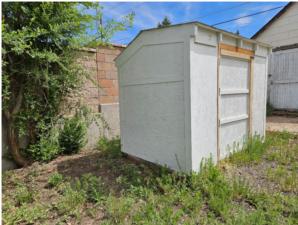
West and south elevations of F4 (shed), view southeast (Roll 26-450, image 110100; Emily Wren; 5/22/2026)
