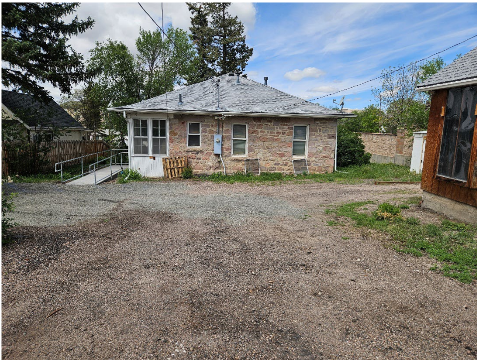
East elevation of the residence, view west (Roll 26-450, image 110234; Emily Wren; 5/22/2026)
