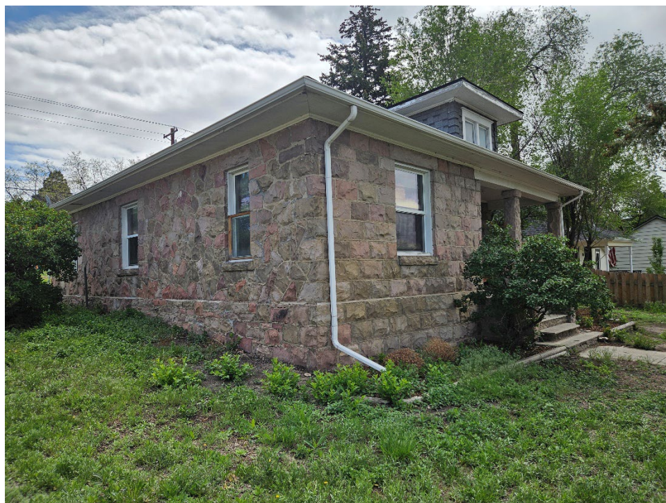
Primary (west) and north elevations of the residence, view southeast (Roll 26-450, image 110315; Emily Wren; 5/22/2026)
