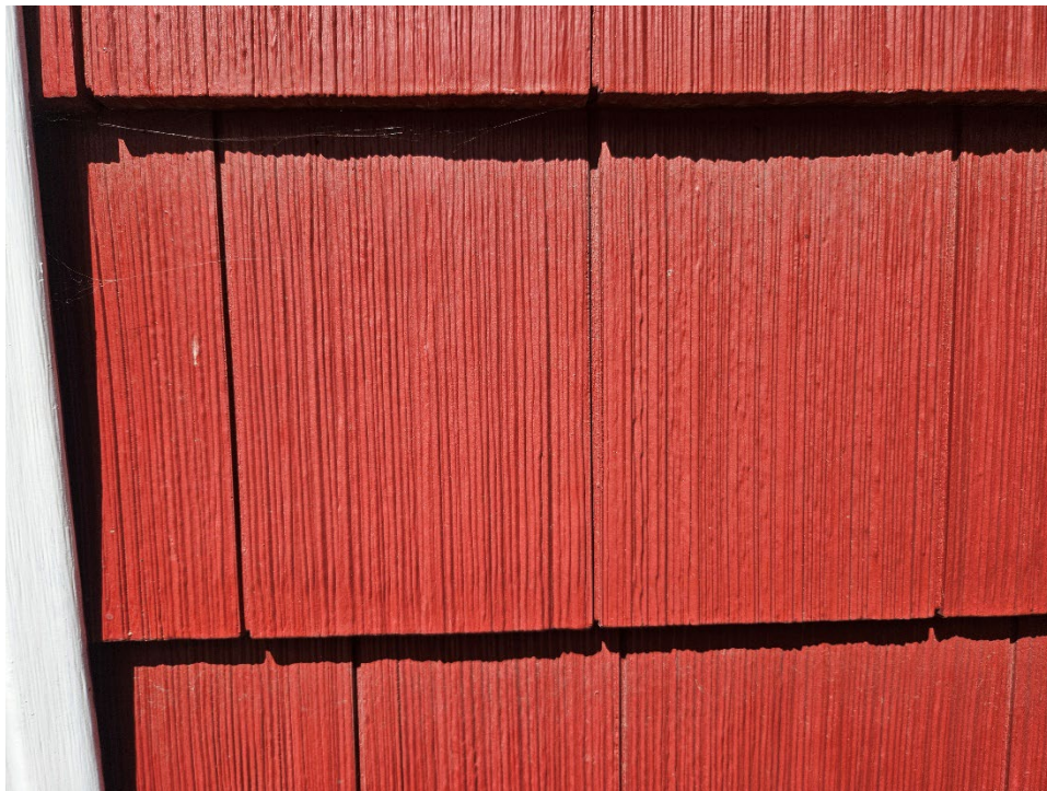
Close-up of the replacement shingle siding
