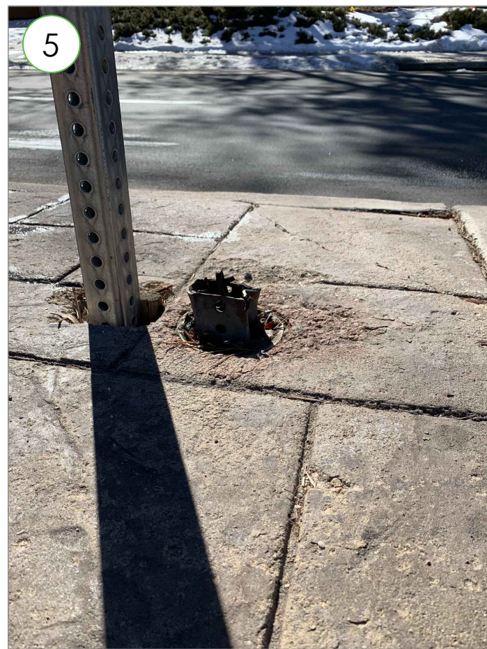
VIEW LOOKING AT EXISTING SIGNAGE POST.
