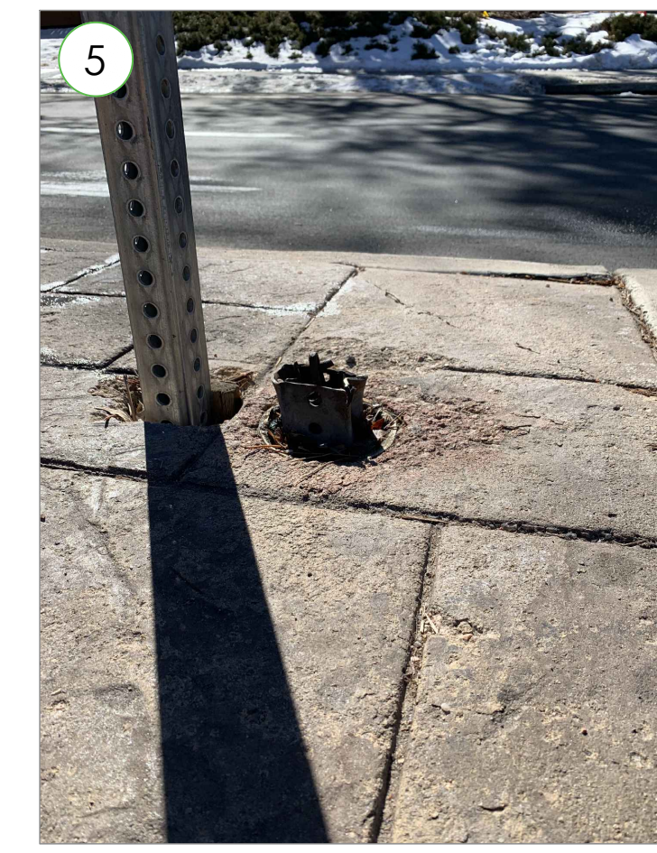
VIEW LOOKING AT EXISTING SIGNAGE POST.
