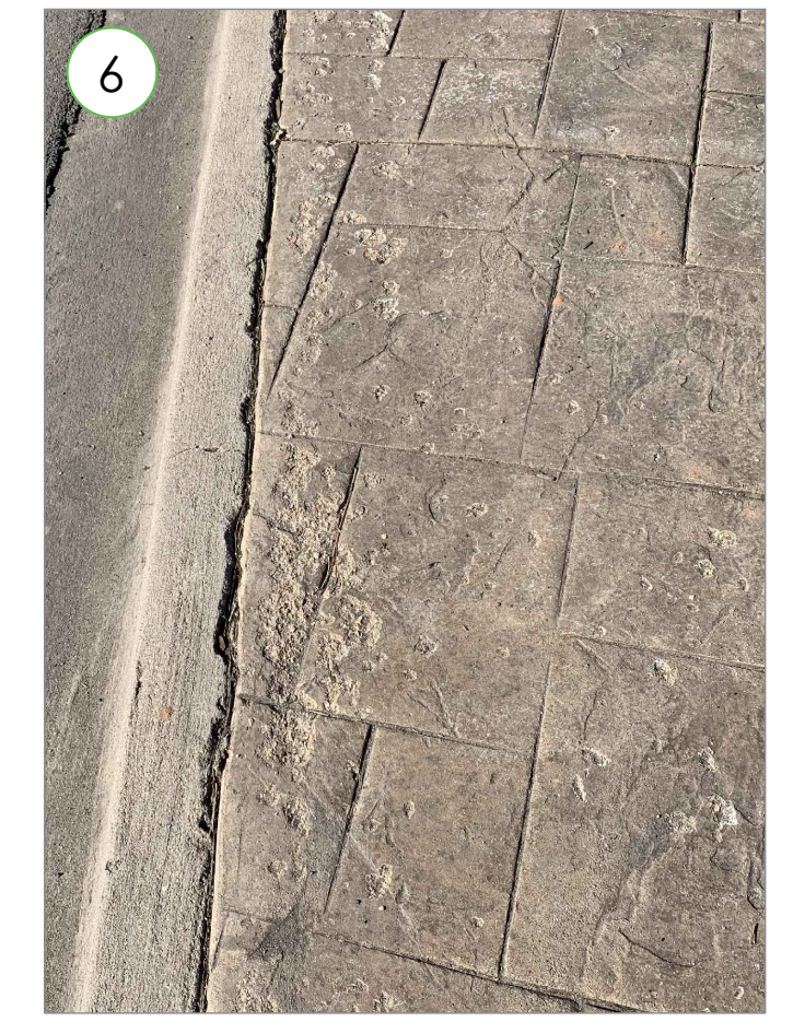
VIEW LOOKING AT FLECKING/ SPALDING OF EXISTING STAMPED/COLORED CONCRETE.
