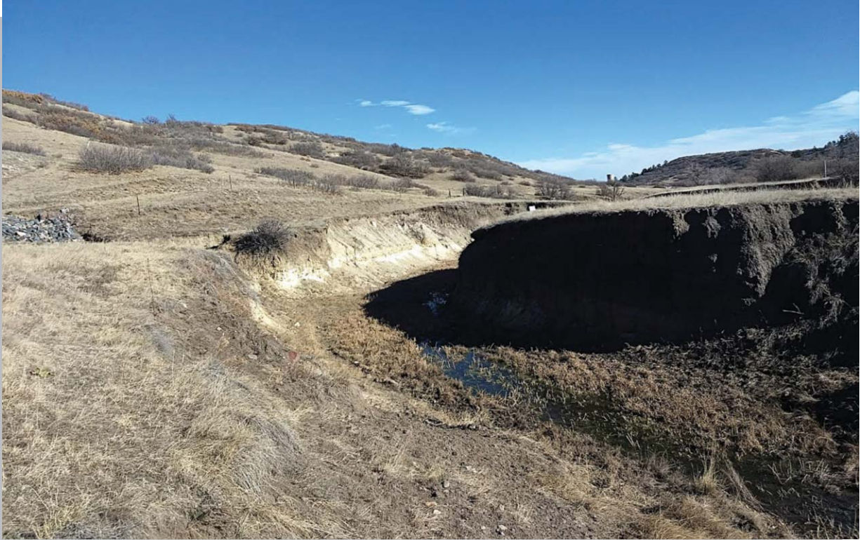
Photo 9 - A section of Scott Gulch showing channel and bank degradation following the 2013 floods. View is to the east.
