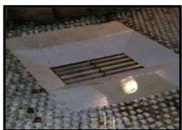
CDOT Type D Inlet Parallel (Flat & Depressed)
